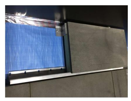
41) The top course below an eave or soffit requires brackets to be used in vertical joints.
