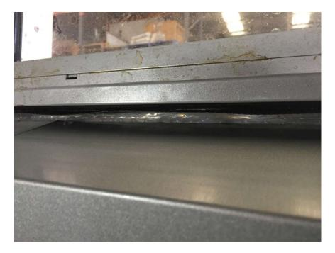
48) When applying sealant, it is advisable to protect the sill to ensure it is not accidentally marked.
