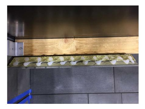
55) Prior to installation of the vertical adjoining piece a bracket is fitted into the locating groove. A tip is to ensure you have your fixing ready to go before you place the block.
