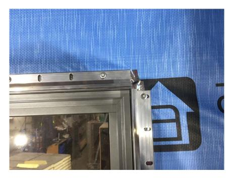
26) There a block runs below a window is should be cut to fit underneath the Reveal extrusion that will support the sill. A groove must be cut into the vertical part of the cut to accept the locating flange on the Reveal extrusion that runs up the side of the window.
