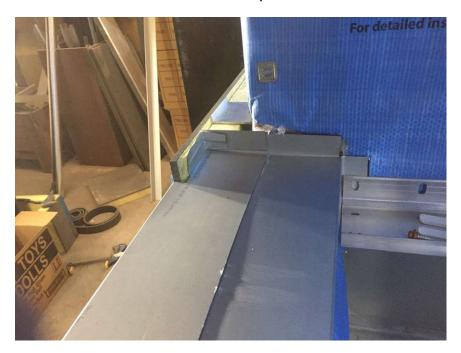
22) Flashing should be taped to sarking to ensure water tightness.
