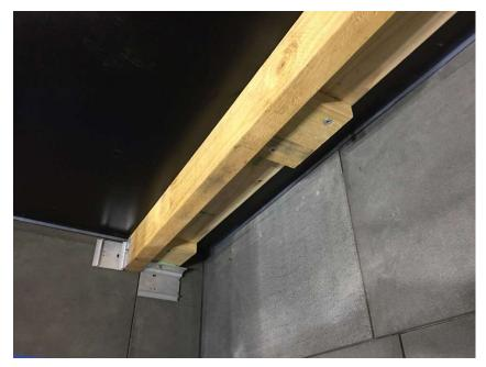
51) Once a block is cut to produce the same 'quirk mitre' detail as described previously along one edge a bracket is pushed into the locating groove prior to installation.
