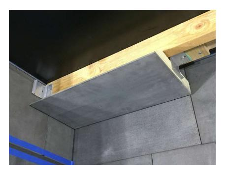
53) It is useful to mark the line of the soffit and vertical elements to help positioning of the brackets.
