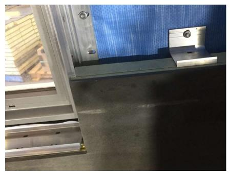
30) Tape should be applied to the top edge of the Reveal extrusion that forms the lintel, and the junction between the vertical and horizontal Reveal extrusions sealed with silicone.
