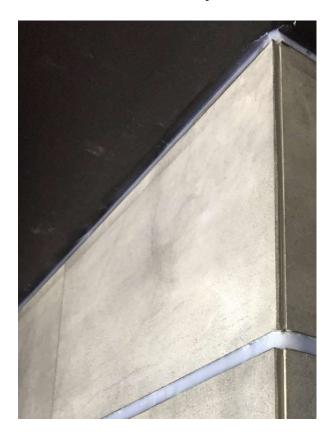
The product is weatherproof if installed according to the above instructions, even though the nominal 3mm joint will appear to be open once finished. This 'open' joint may be caulked or grouted in a complementary colour once the wall is finished without affecting its performance. Should a traditional 'mortar joint' be desired a bevel is machined on the blocks and flexible sanded grout used to fill the joint, giving it the appearance of having been laid with mortar as seen below.
