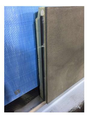
8) Clips are fixed at maximum 600mm centres and joiner extrusions placed in horizontal joints.
