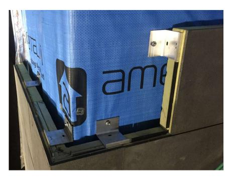
38) It may be necessary to provide nogging at the back of stud walls to take the brackets set in vertical joints. Be careful to ensure they are at a height that will allow for the brackets to be fixed without extending above the top of the blocks. The black marks seen in the image below are 60mm below the height of the horizontal expansion joint. Additional nogging has also been placed below the top plate to take vertical brackets below the eave lining.
