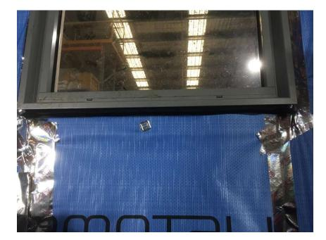
5) All joints in sarking should be lapped a minimum of 50mm and taped.
