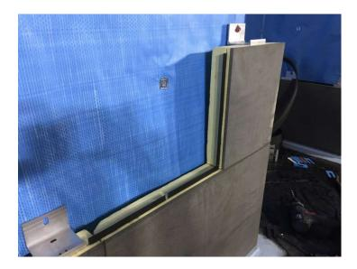
16) A helpful tip is to 'dry lay' each block before applying sealant. This helps ensure a proper fit before sealant is used, and adjustments can be made if necessary without creating mess. It is important to avoid having the sealant contacting the face, particularly for darker coloured stones. Note below how a mark has been made where the dry laid block finished which gives a guide to where the sealant should stop before the block is laid.
