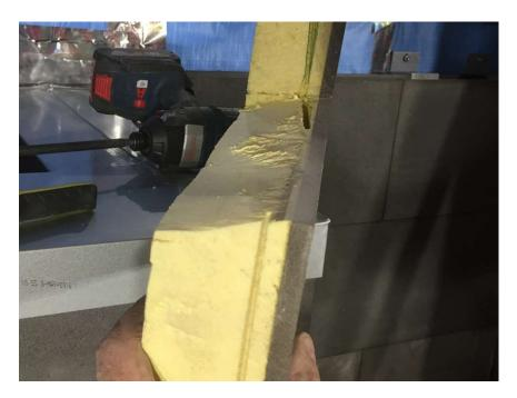
28) Tilting the top of the block forward, place the block on the locating groove below and push down to height before standing block up to ensure it is in line with the vertical wall face.
