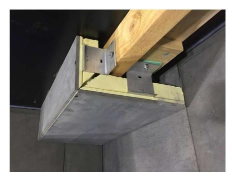
57) It is best to leave to last one of the blocks that is towards the centre rather than at the extreme end of the soffit section.
