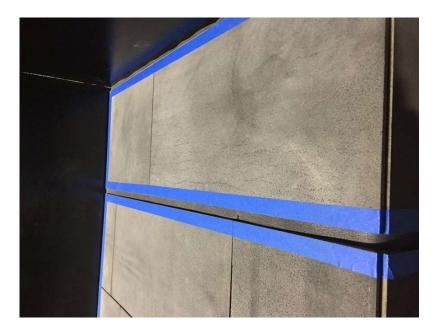
44) Sills come with a locating groove that ensures it cannot come loose once installed. The groove allows the sill to lock onto the locating flange on the Reveal extrusion. The sill may also have a 'drip-line' cut approximately 15mm back from the front edge either in the factory or done on site.
